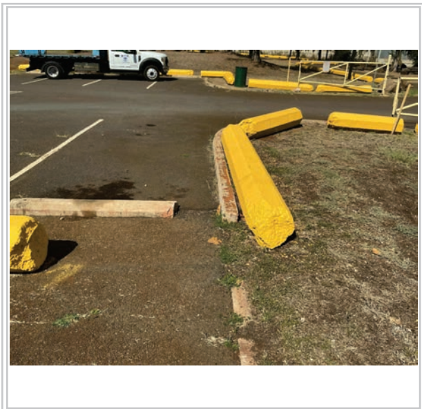
Area to be repaved
