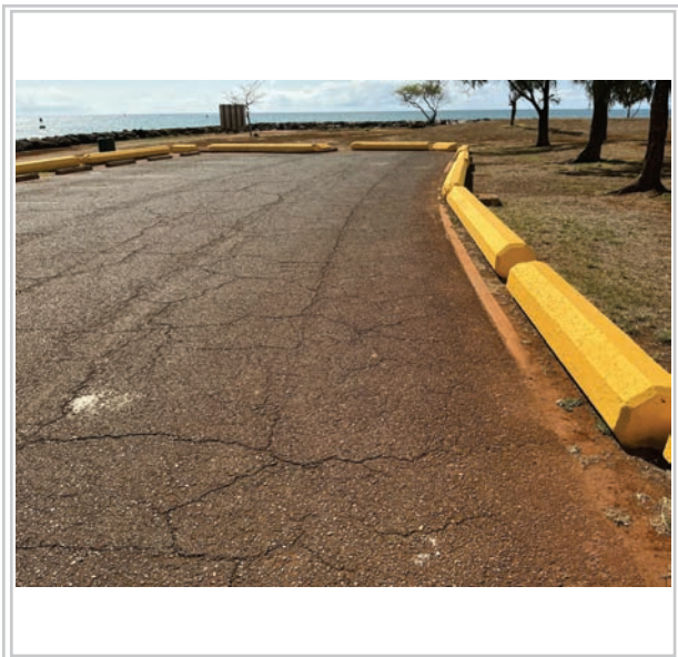
Area to be repaved
