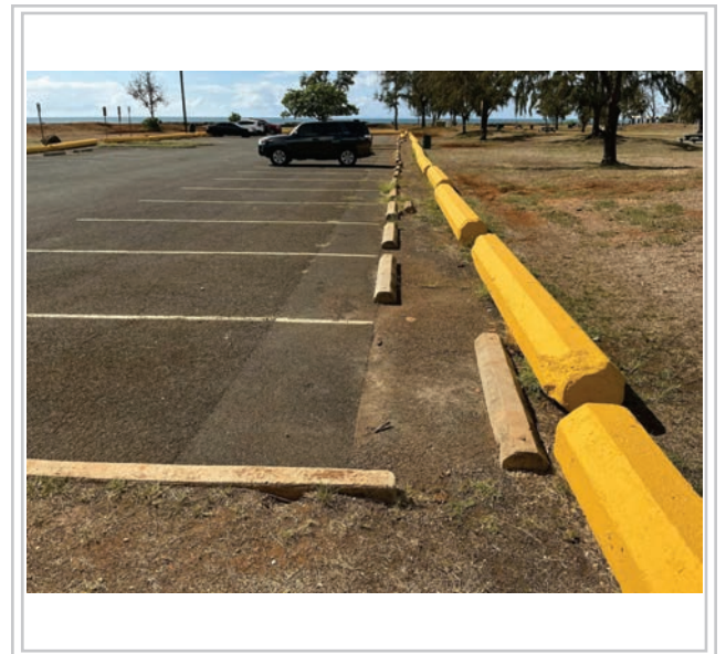
Area to be repaved
