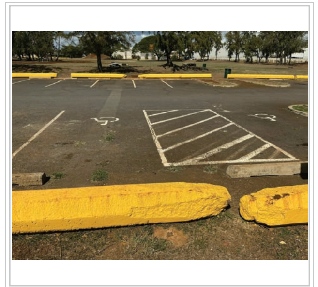
Area to be repaved
