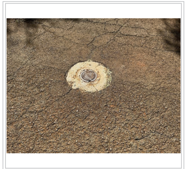
Area to be repaved
