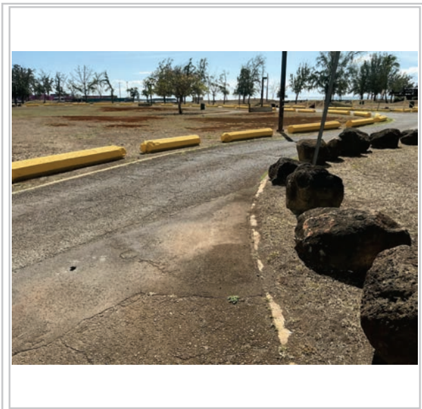
Area to be repaved
