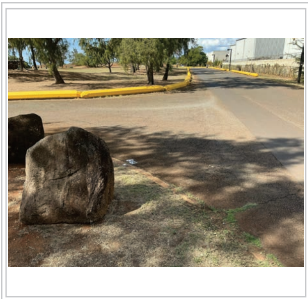
Area to be repaved
