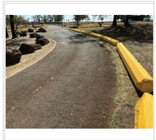
Area to be repaved
