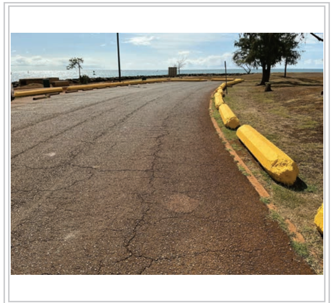
Area to be repaved
