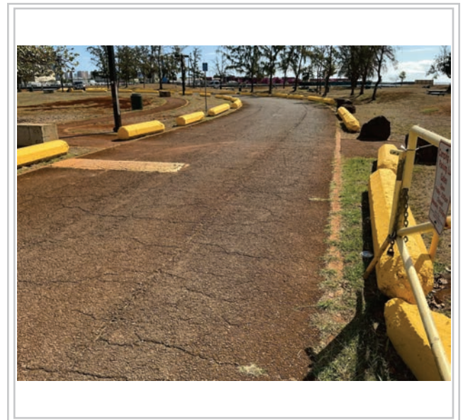
Area to be repaved
